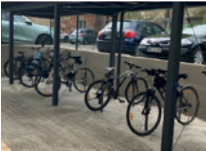
Finalized bike-storage facility
