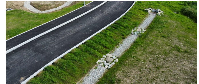
Bioswale via Ari, Besozzo (Regione Lombardia, Italy). Design and construction supervision by IRIDRA – under construction
