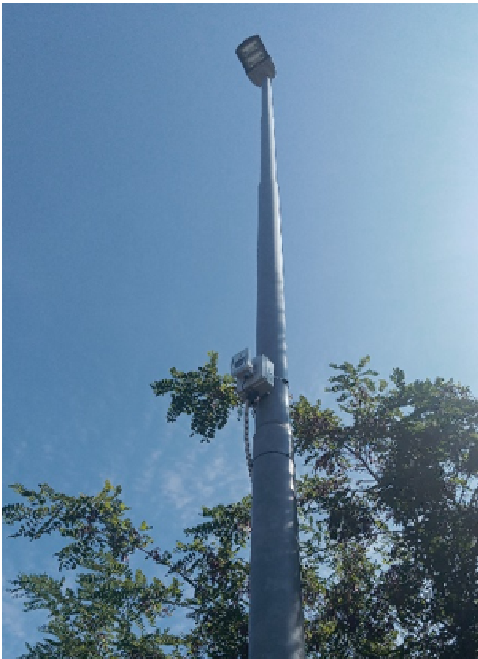
Traffic & Air-Quality Sensor Network in Nova Gorica-Gorizia: Teleram S2 – Outdoor module
