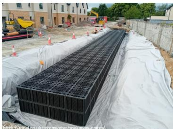
https://trical.co.uk/stormwater/soakaway-crates/ Geocellular soakaway crate system at Residential development in Killarney (Ireland)
