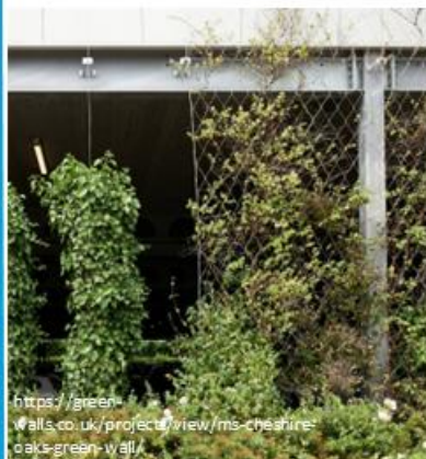
Green wall at the McArthurGlen Designer Outlet Cheshire Oaks in Ellesmere Port, UK, constructed using modular GSKy planter units.
