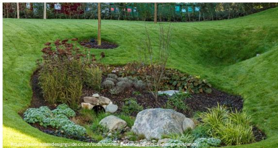
Bioretention area in Temple Farm, Chelmsford (UK)
