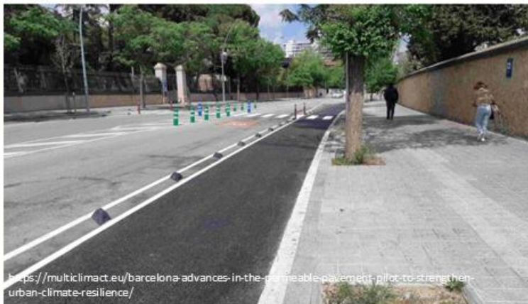
Permeable pavement installation in Barcelona (Spain)
