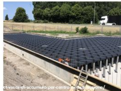
Installation of Atlantis Tank underground retention system for the Zaandam Distribution Centre project, Netherlands
