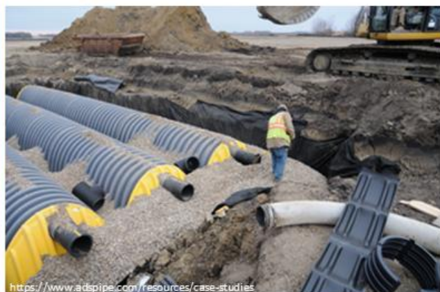
Plastic stormwater chamber system installed at the Prinsburg yard expansion in Minnesota (USA) for underground stormwater detention and controlled infiltration.
