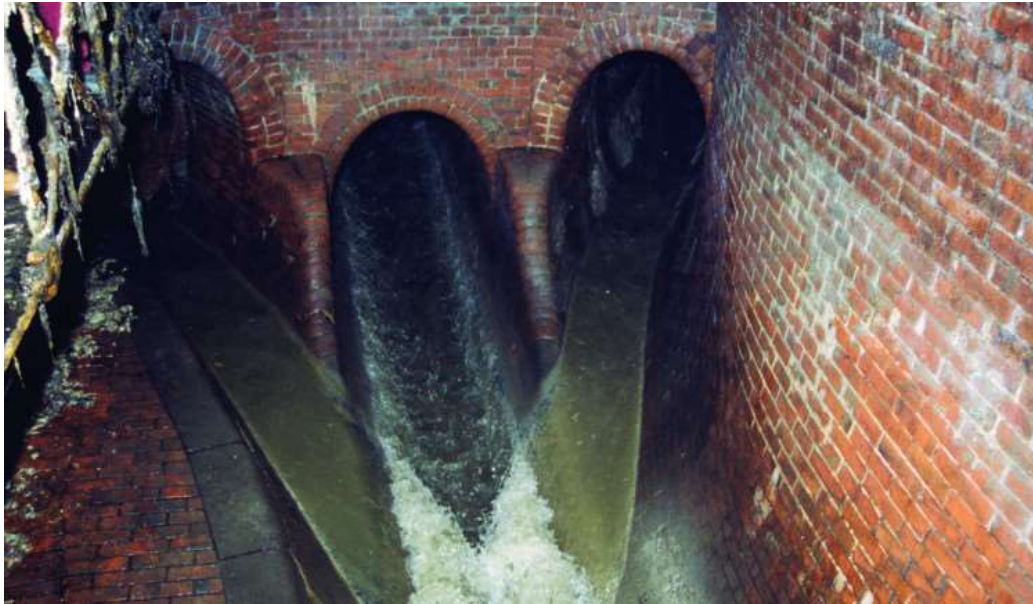
Figure 4: Historic sewer in Prague
