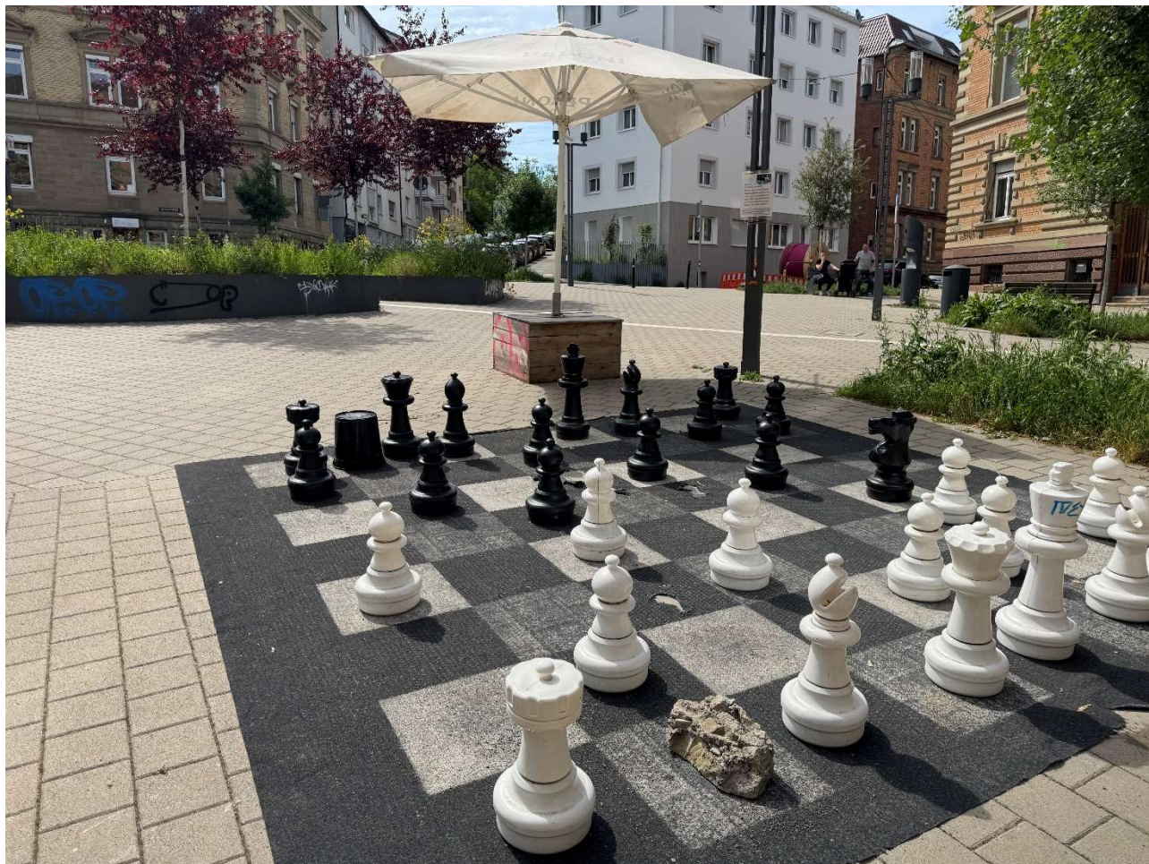
Unsealing and installation of permeable paving with full water- and air-permeability at Schützenplatz in Stuttgart.
