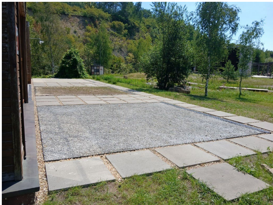
Photo 2: Pilot installation in Jaworzno - permeable surfaces: cavernous concrete, geogrid and mineral-resin pavement.
