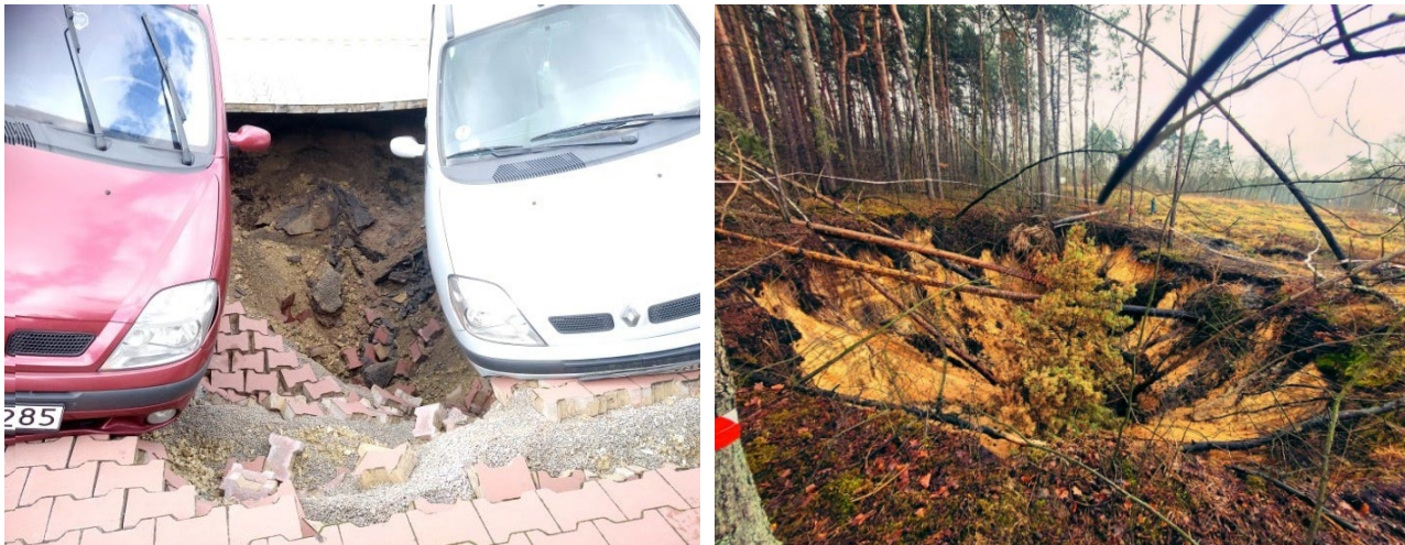
Photo 1: Examples of land subsidence problem in Jaworzno, Poland
