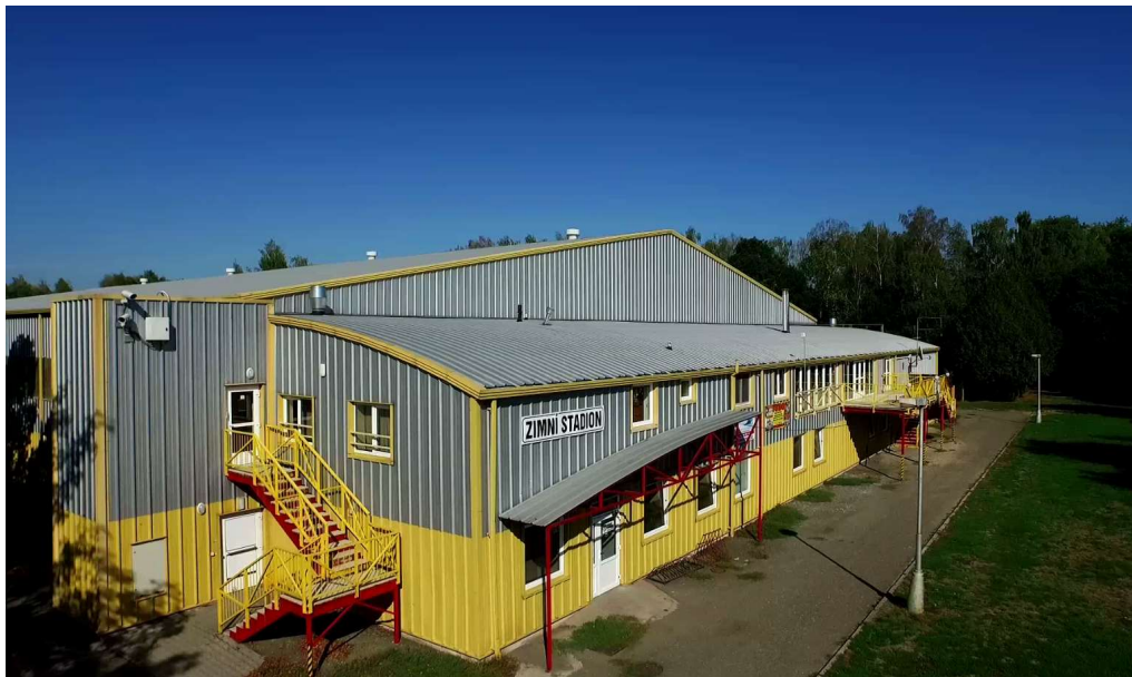
Figure No.5: Winter Stadium Building
