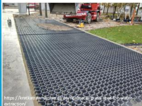
Grass grid permeable pavement installed around a groundwater abstraction facility in Golina near Jarocin (Poland).
