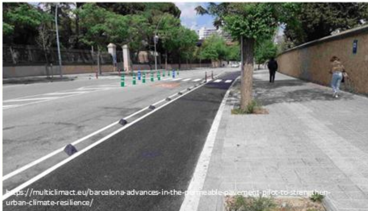
Permeable pavement installation in Barcelona (Spain)
