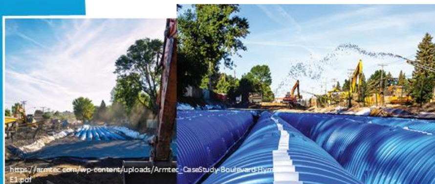
Plastic stormwater chamber system installed beneath a bicycle path along Boulevard Hymus in Pointe-Claire (Canada) for underground stormwater detention.
