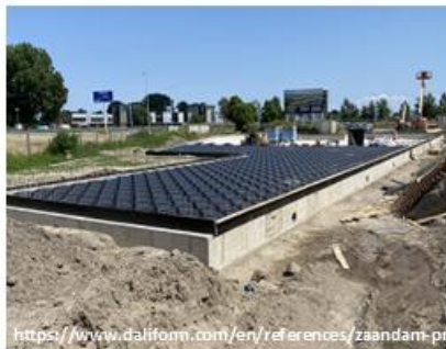
Installation of Atlantis Tank underground retention system for the Zaandam Distribution Centre project, Netherlands
