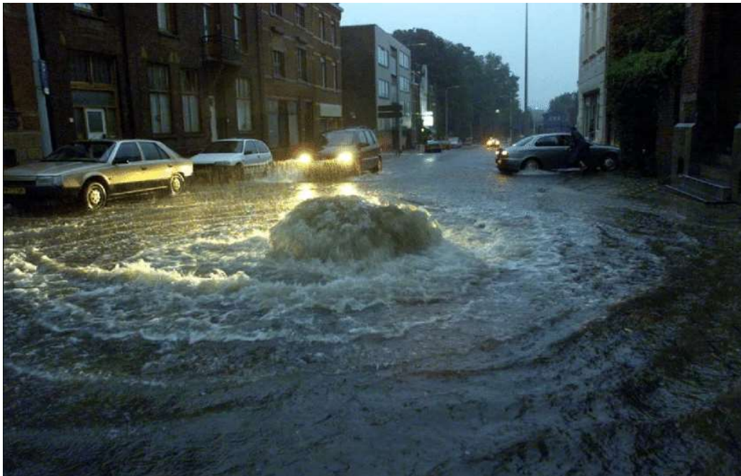
Figure 3: Overloaded sewer system during heavy rains (Kluck et al, 2005)
