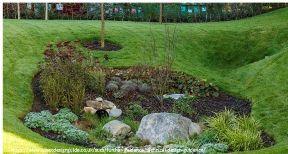
Bioretention area in Temple Farm, Chelmsford (UK)
