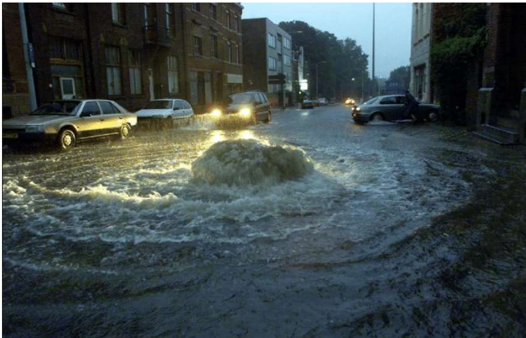
Figure 2: Overloaded sewer system during heavy rains (Kluck et al, 2005)
