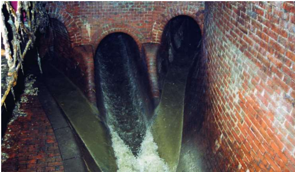
Figure 4: Historic sewer in Prague
