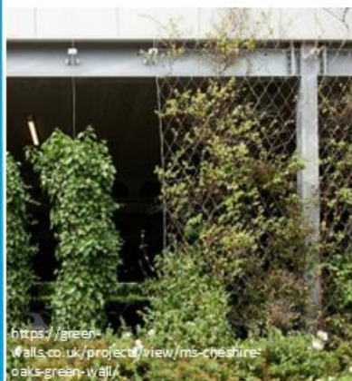
Green wall at the McArthurGlen Designer Outlet Cheshire Oaks in Ellesmere Port, UK, constructed using modular GSky planter units.
