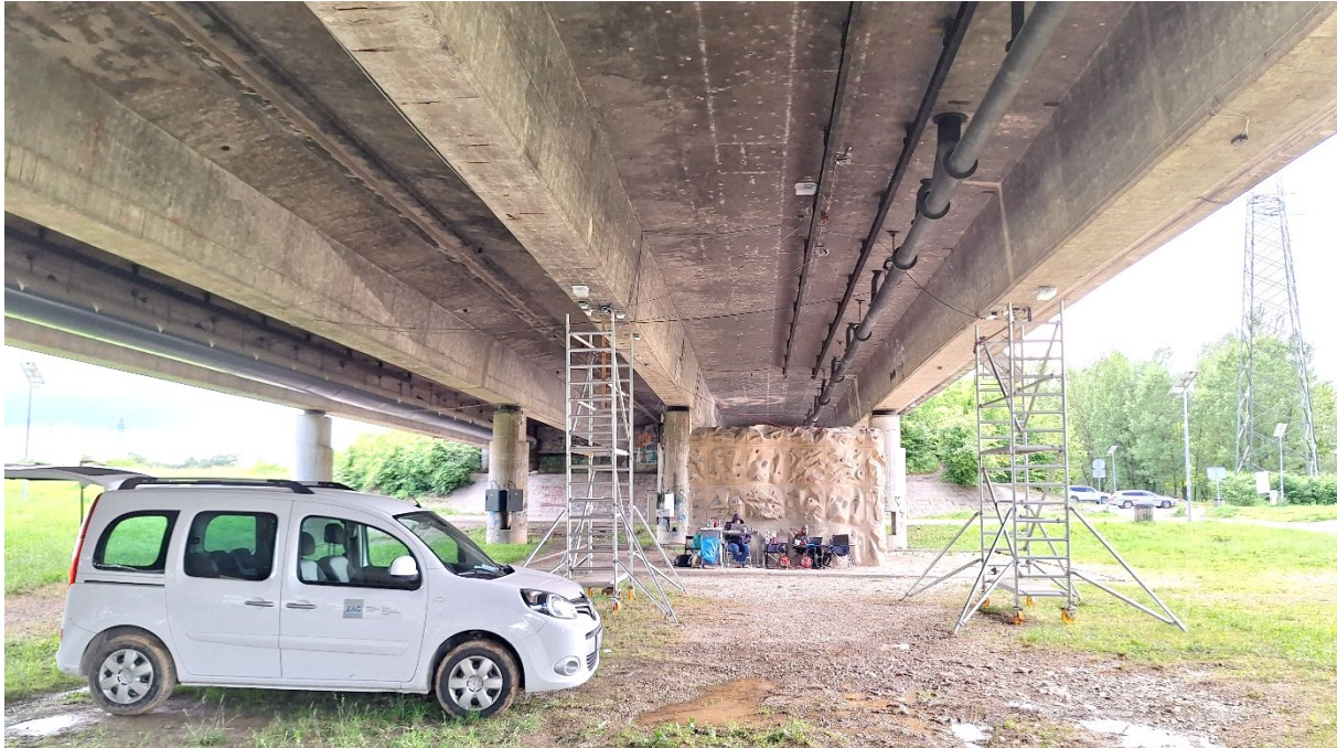
Figure 6. View under the superstructure of the Tomačev bridge – view towards Ljubljana
