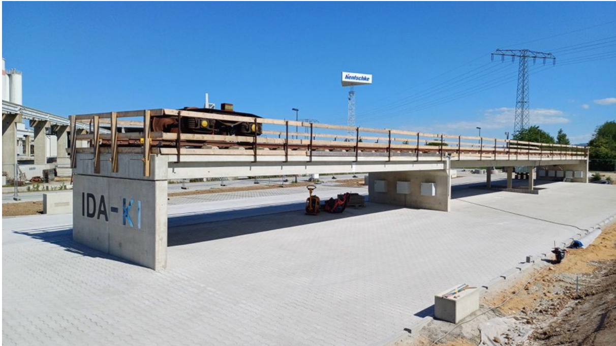
Figure 11. openLAB research bridge
