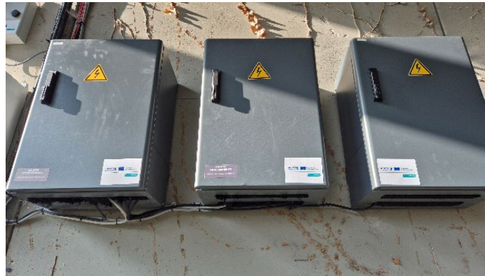
Figure 19. Installation of instrumentation on Sant'Ambrogio bridge
