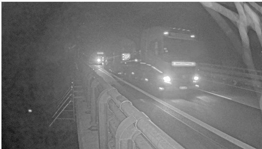
Figure 68. An exceptional transport at Sant'Ambrogio bridge (GVW approx. 80 t)
