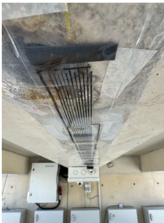
Figure 56. Photo of leakage foil installation on openLAB bridge.
