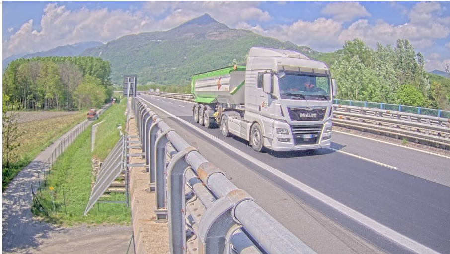
Figure 67. A 5-axle HGV at Sant'Ambrogio bridge (GVW approx. 40 t)
