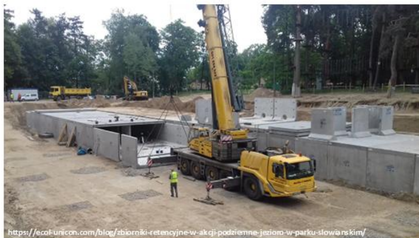
Construction of a underground retention tanks in Park Słowiański in Gorzów Wielkopolski
