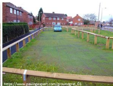
Grass grid permeable pavement installed in Stainforth near Doncaster (United Kingdom) to create off-road parking while maintaining a permeable vegetated surface.
