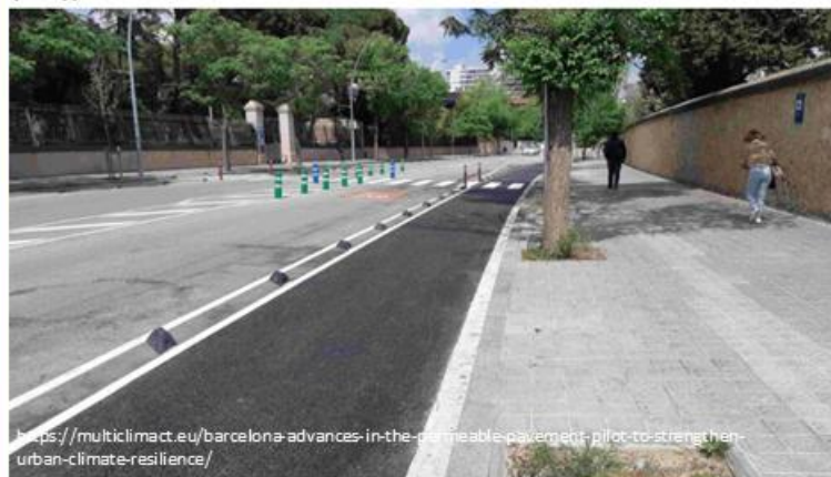
Permeable pavement installation in Barcelona (Spain)
