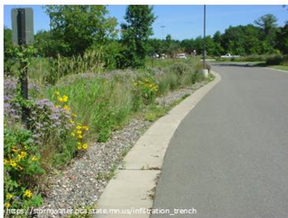
Infiltration trench in Lino Lakes (US)
