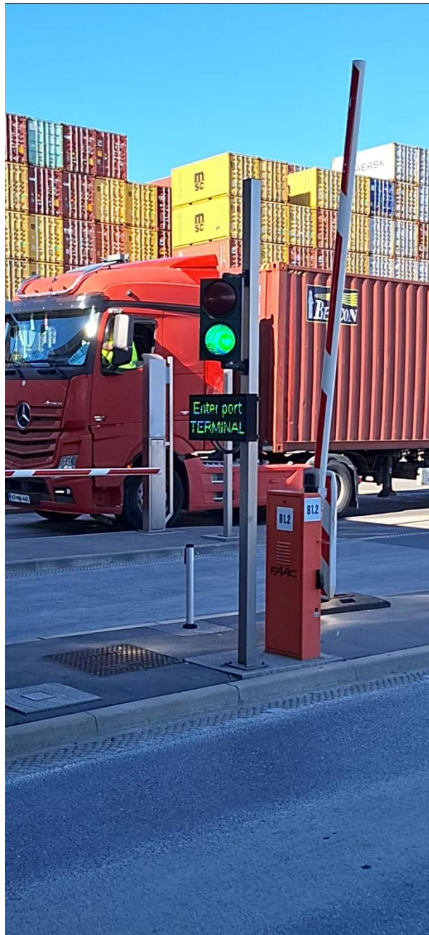
Figure 11 - view of the green light and displayed information after the truck passes through the OCR
