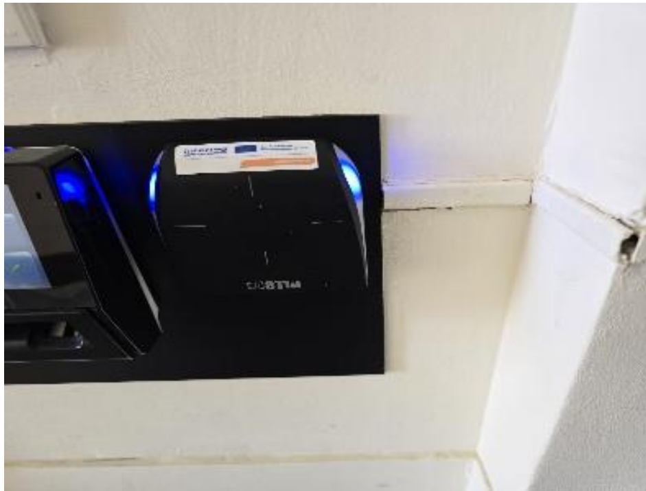
Figure 6 - Equipment installed in the port of Rijeka
