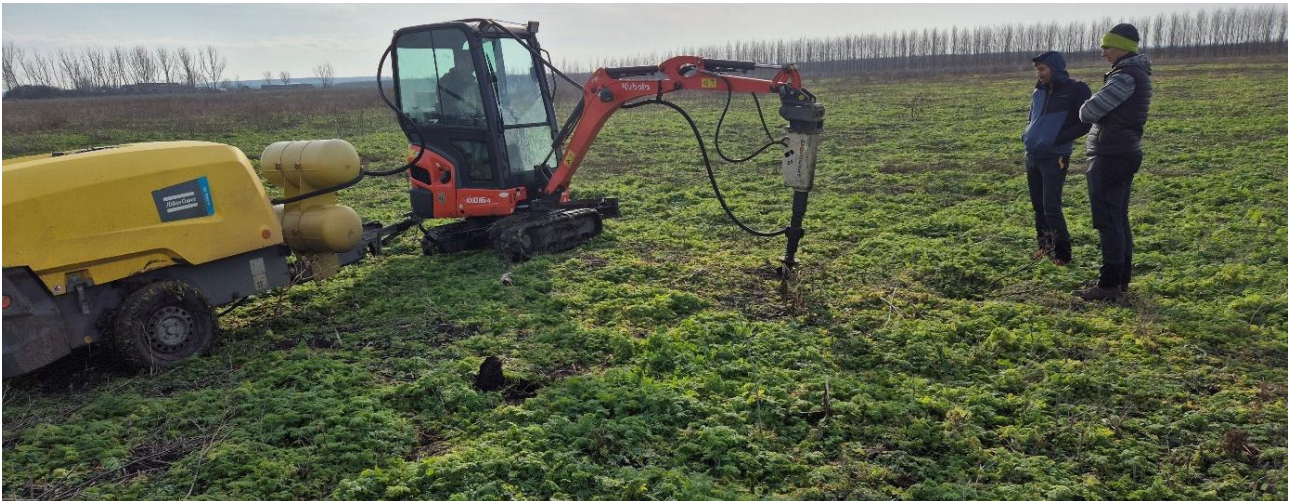
20. Figure: Soil ventilation procedure (12 bar pressed air, 1-1,5 m deep)
