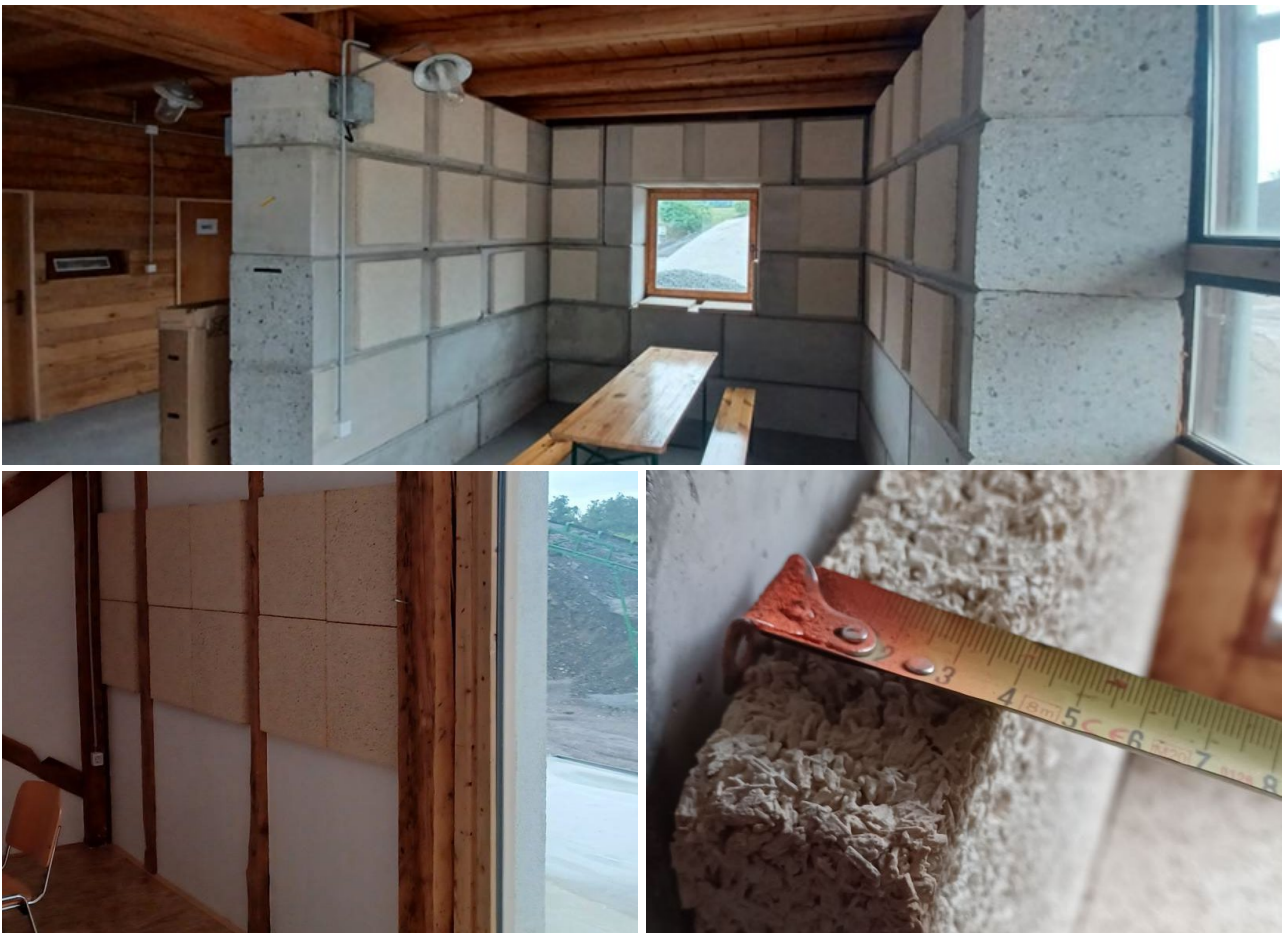
Figure 1: Installed test specimens; top: ground floor with panels mounted individually; bottom-left: 1 st floor panels mounted in batches; bottom-right: panel detail with side exposed
