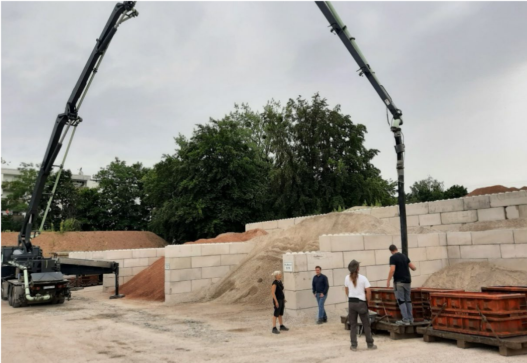
Figure 4: Pumping test on the Bayernkaserne site with 100 % recycled concrete
