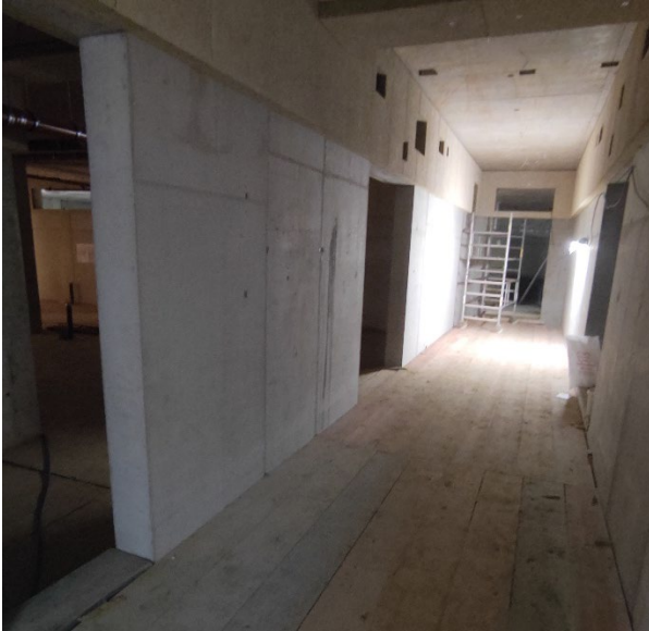
Figure 9: walls in the basement made of recycling concrete with 100% recycled aggregate
