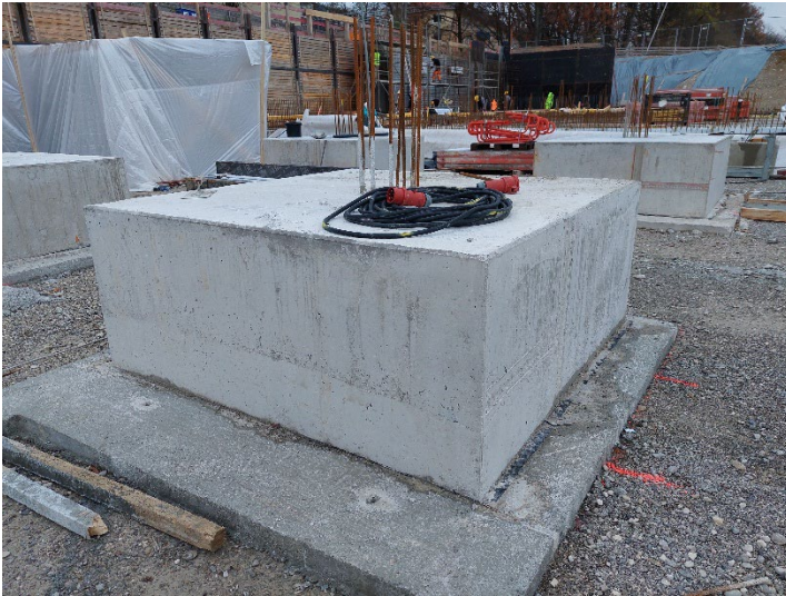
Figure 7: Foundation made of recycling concrete with 100% recycled aggregate
