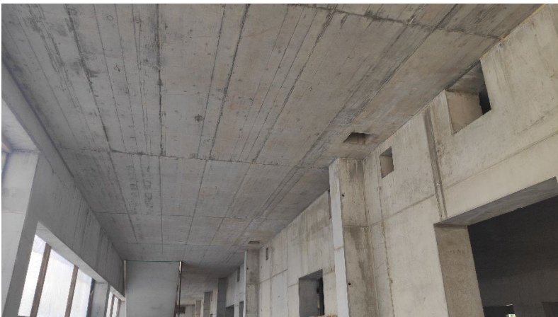
Figure 8: View on the ceiling panel from below made of recycling concrete with 100% recycled aggregate
