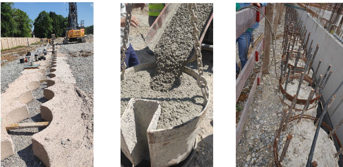
Figure 6: Left: Prepared building site with the drilling template produced with recycling concrete with 100% recycled aggregate; middle: fresh concrete during producing a bore pile with concrete with 100% recycled aggregate; right: hardened borepiles
