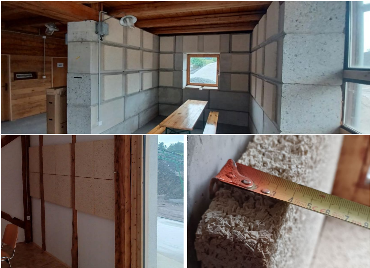
Figure 2: Installed test specimens; top: ground floor with panels mounted individually; bottom-left: 1 st floor panels mounted in batches; bottom-right: panel detail with side exposed
