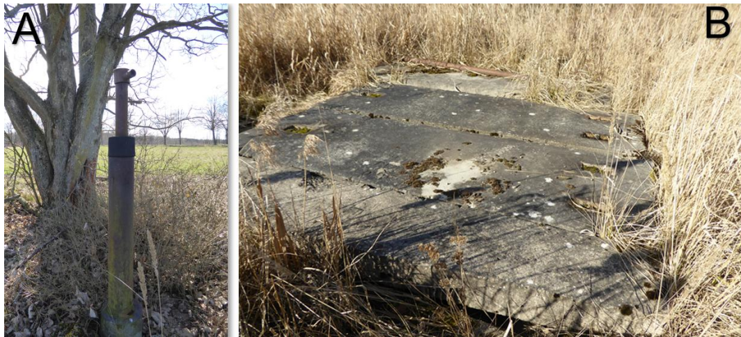
Figure B.2: Rests of (a) old copper well and hydrocarbon well (b) in the Lausitz region. Source: LBGR field survey, 2025.
