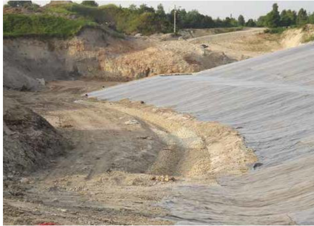
Figure 14. Bentomat insulation of the slopes of the internal dump
