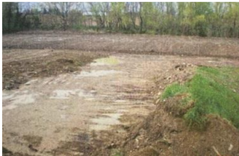
Figure 4. Covering with geotextile and soil (about 30 cm) in 2009-2010. Source [2]
