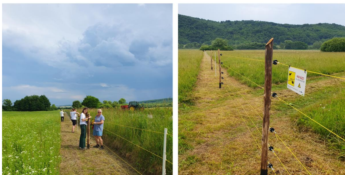
Figure 33.: The installation of the predator-proof electric fence in Dövény, HU by volunteers (photos © WWF HU).
