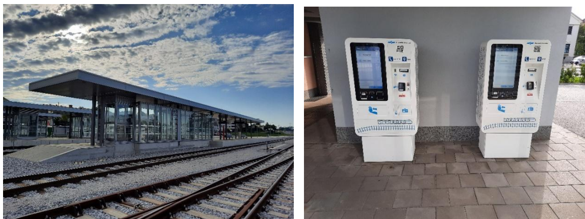
Figure 8: Grosuplje railway station & ticket vending machines
