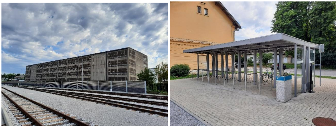
Figure 10: Grosuplje P+R garage at railway/bus station & bicycle shelter next to the garage
