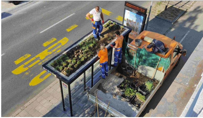
Installation of green roof on bus stop
