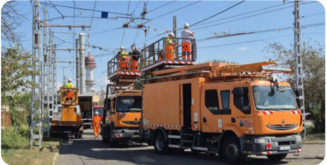
Figure 24: Installation of a trolleybus switch by the SZKT maintenance team.
