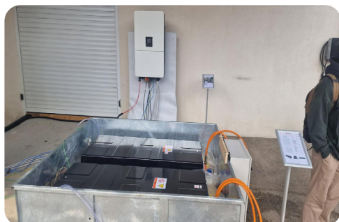
Figure 27: Key components of the BESS system: PV panels, inverter and second-life battery pack.
