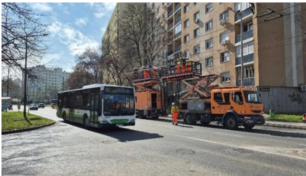
Figure 3 Installation of new trolleybus switches
