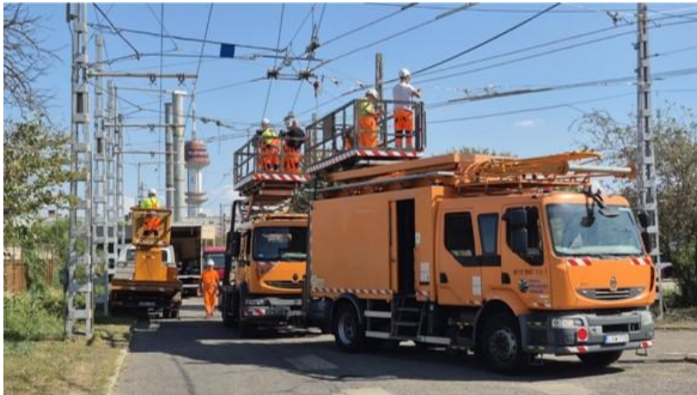
Figure 4 Installation of new trolleybus switches
