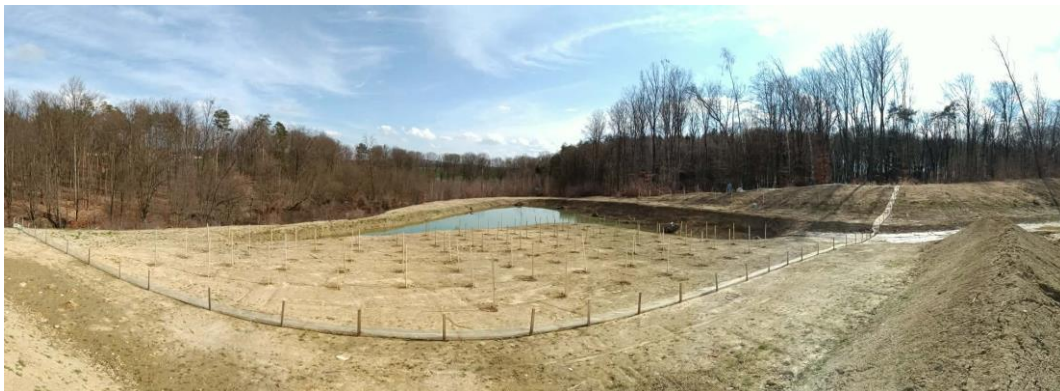
Figure 3. View of the planting area from the opposite side.
