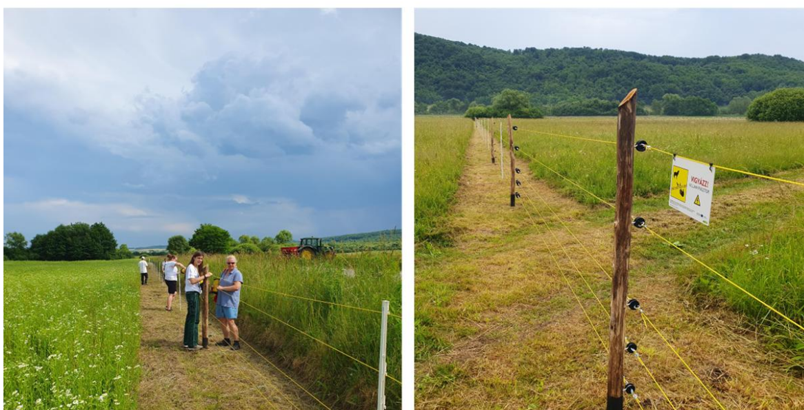
Figure 33.: The installation of the predator-proof electric fence in Dövény, HU by volunteers (photos © WWF HU).
