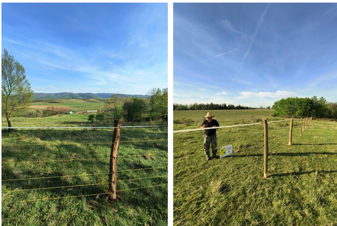
Figure 28.: Predator-proof electric fence installed in Nekézseny, HU (photo © WWF HU).
