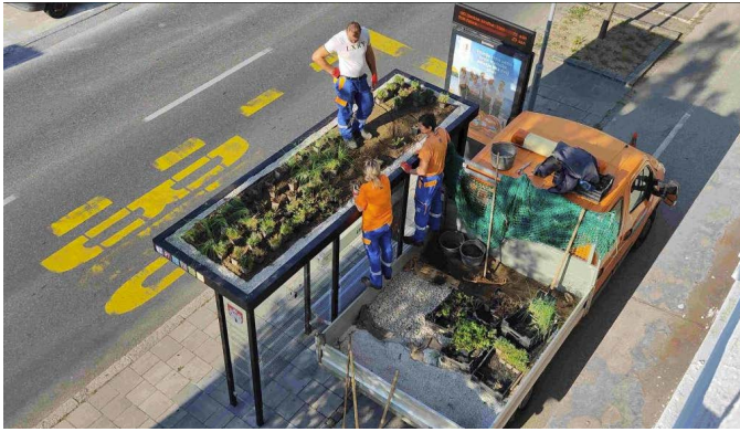
Installation of green roof on bus stop
