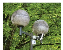
Climate sensors installed on street lamps
