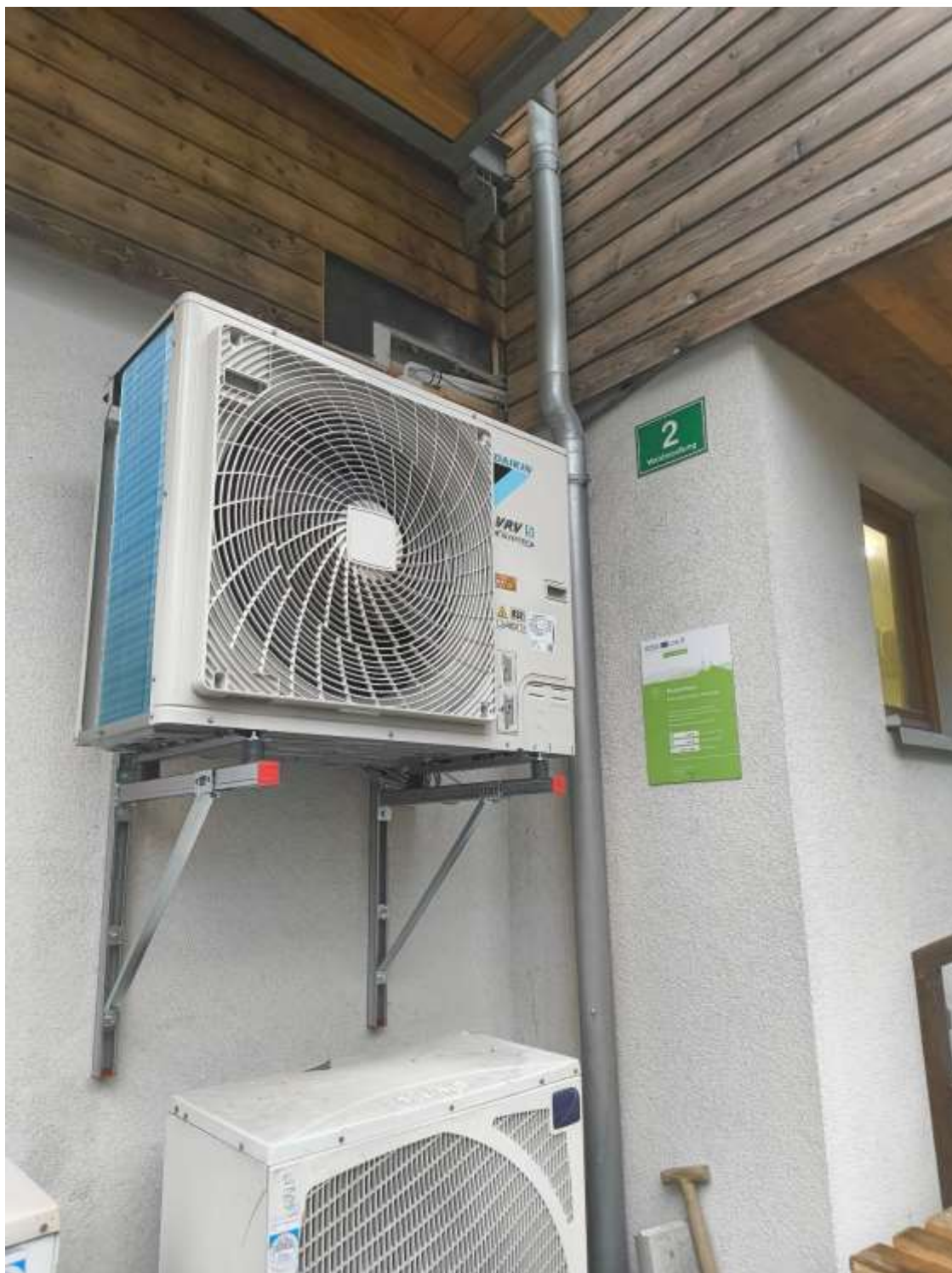
Outdoor unit of air condition
