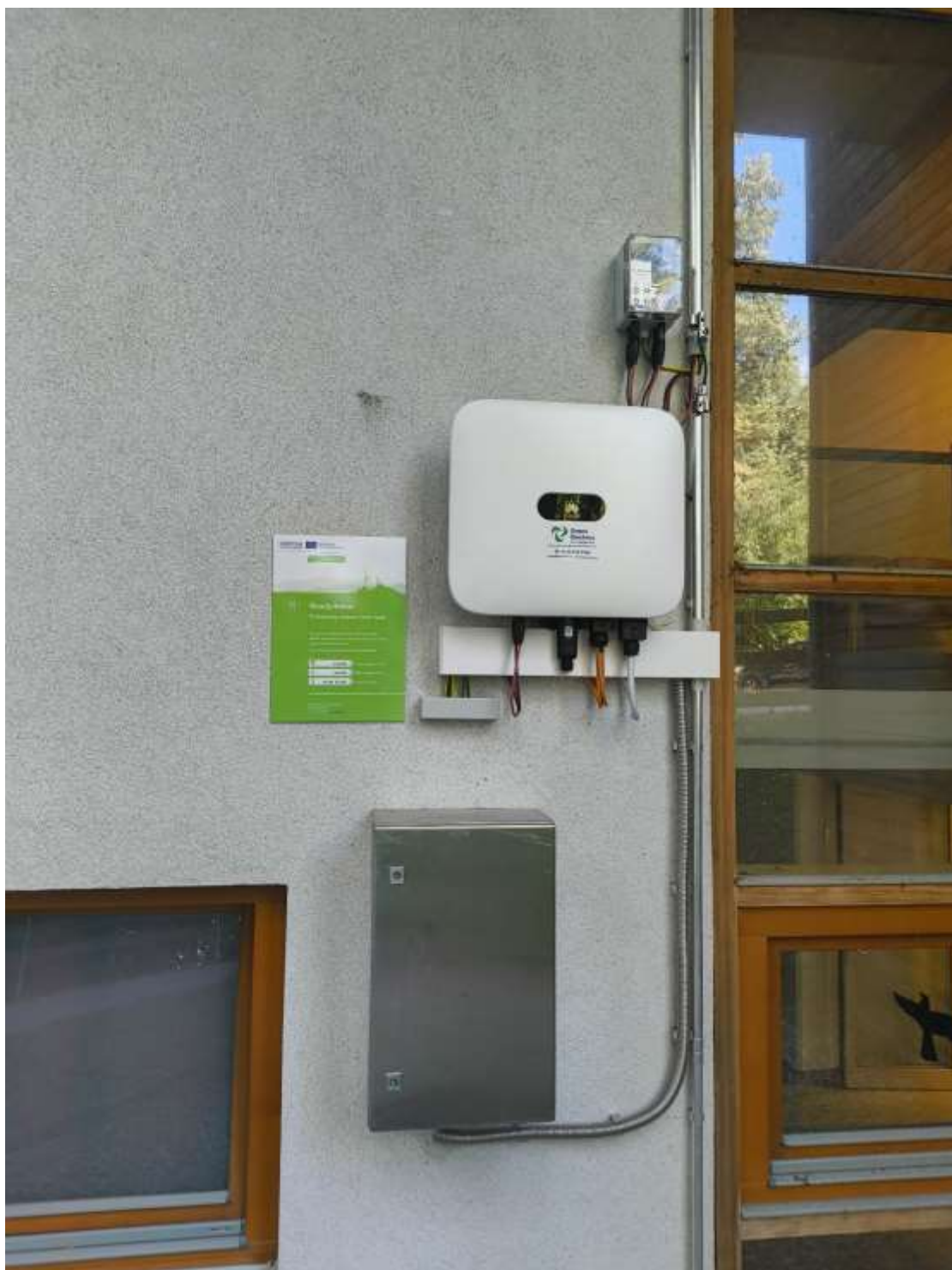
Inverter of PV system
