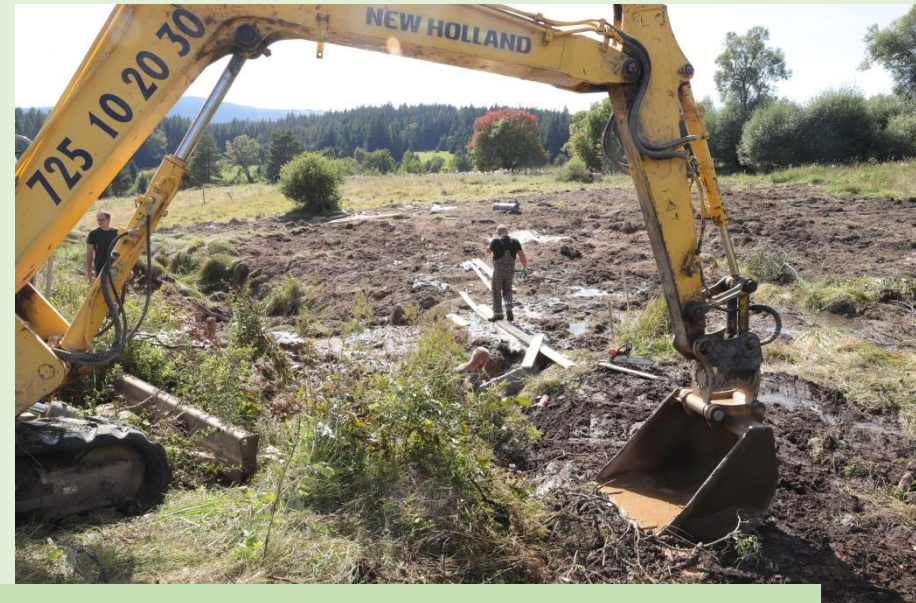
Blocking of drainage ditches by woody dams, infilling of large pits from bank soil deposits
