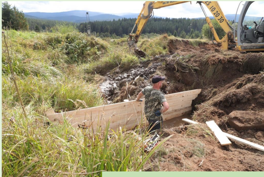
Blocking of drainage ditches by woody dams, infilling of large pits from bank soil deposits
