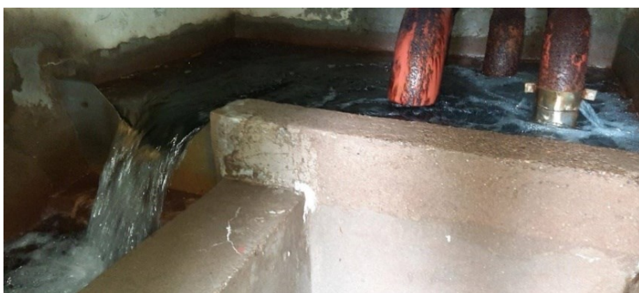
Fig. 41 - Example of captured spring feeding the Toano aqueduct.
