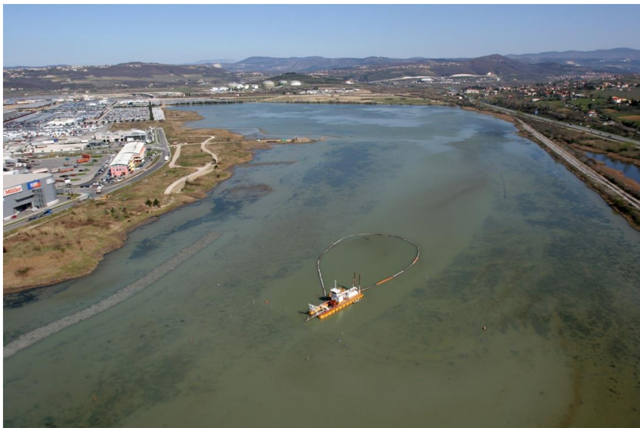
Removal of sediment and deepening of channels in the brackish lagoon in 2007 (NRSZ Archive).
