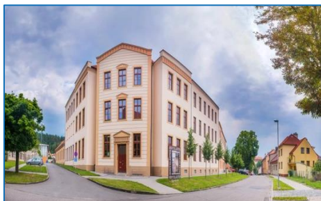
Photo 1 – overall view of the building
