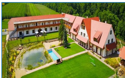
Photo 1 – overall view of the building
