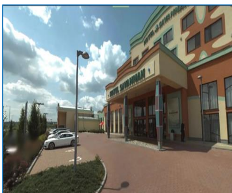
Photo 1 – view of the parking
