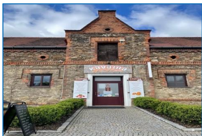
Photo 1 – overall view of the building
