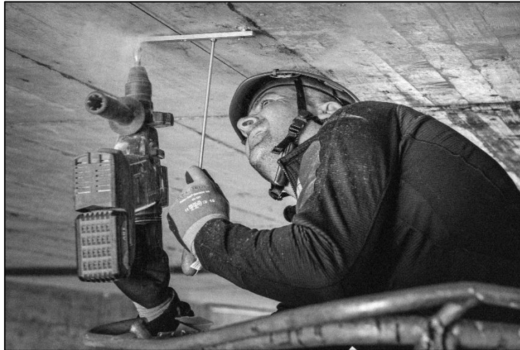
Figure 6: Installation procedure, ST-504 sensors (Source: Cestel).
