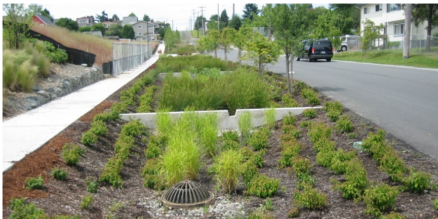
Figure 2. Bioswale along the road (© Rich Blankenship, www.holemanlandscape.com , 2015)
