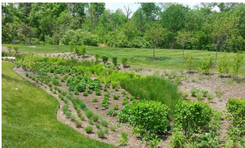
Figure 4. Bioritention basin (© Bluegrass Landscaping & Maintenance, 2018)
