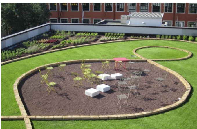
Figure 14. Extensive and intensive green roof (© Tiziana Monterisi)
