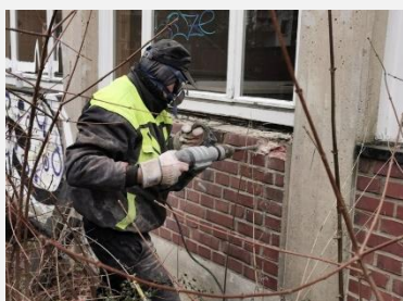
Figure 22 Reuse of old brick in new facade in Aachen. Source: Concular GmbH
