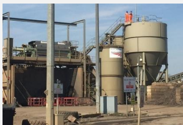
Figure 20 Whitemoor facility. Source: Source: Network Rail (2019)
