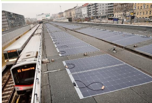
Figure 16. Solar panels at Vienna metro station. Source:
