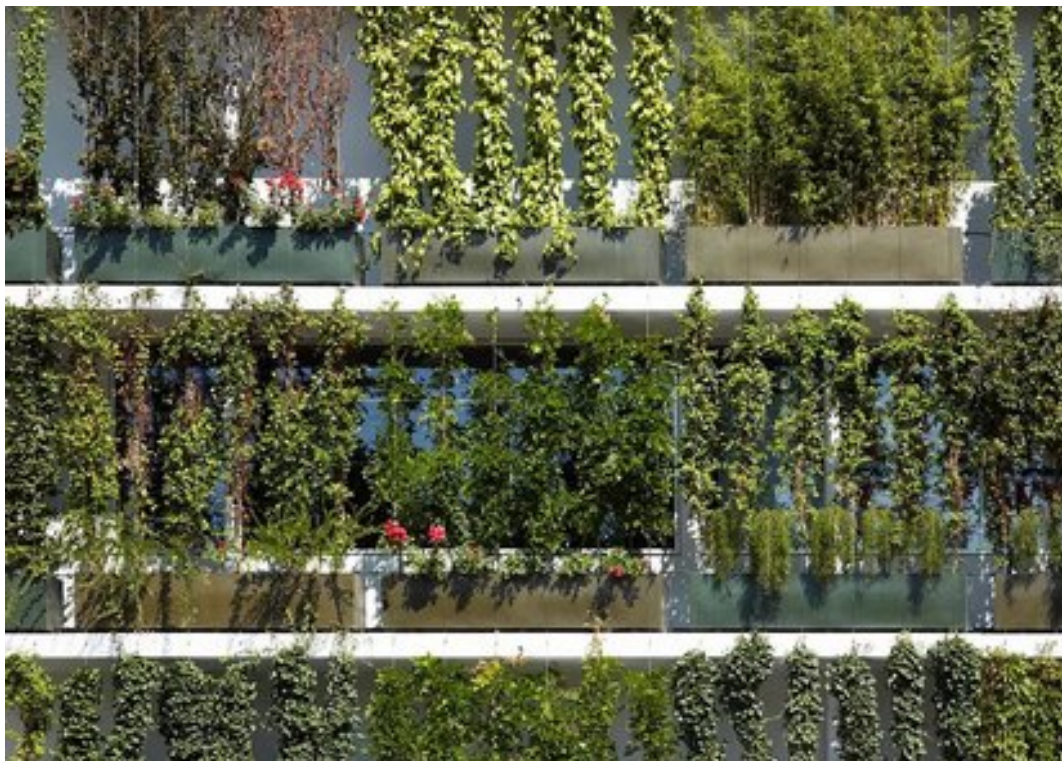
Building shaded with a wire running system
