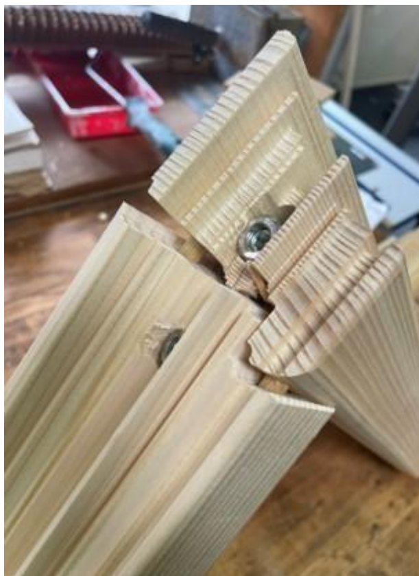
Figure 2: Window frames pre-designed to be easily removed, dissembled and reused.
