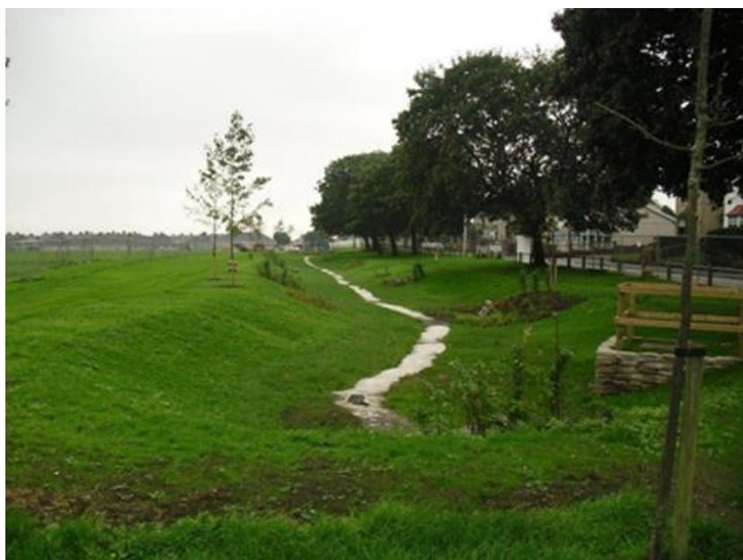
Figure 36: Bioswale Queen Mary's Walk, Llanelli 50
