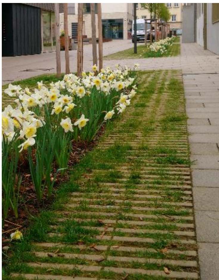
Figure 19: Permeable paving system in Stuttgart, Germany 32
