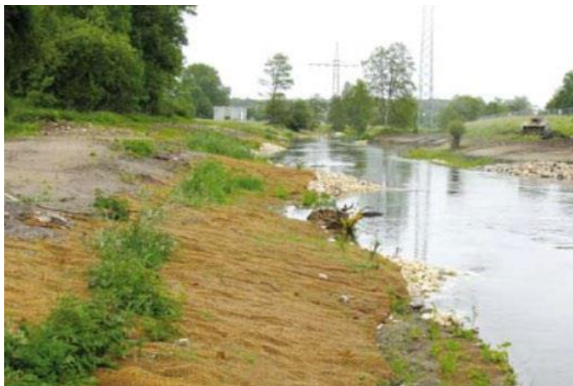
Figure 52: Planted embankment mat 66
