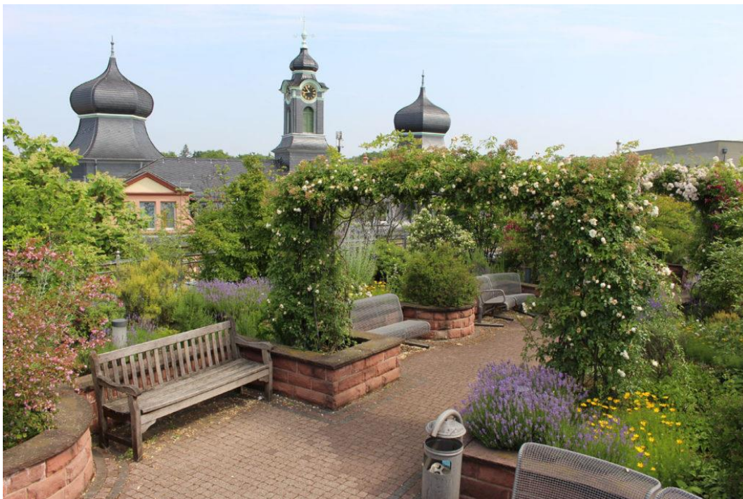
Figure 31: Intensive Green Roof on Bürgerhospital, Frankfurt 43
