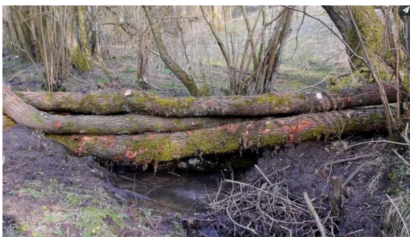
Figure 54: Stroud Rural Sustainable Drainage Project 68
