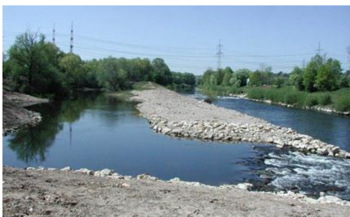
Figure 50: New created branch for water retention, Neckar in Wernau/Neckar ( www.pfrommer-roeder.de )
