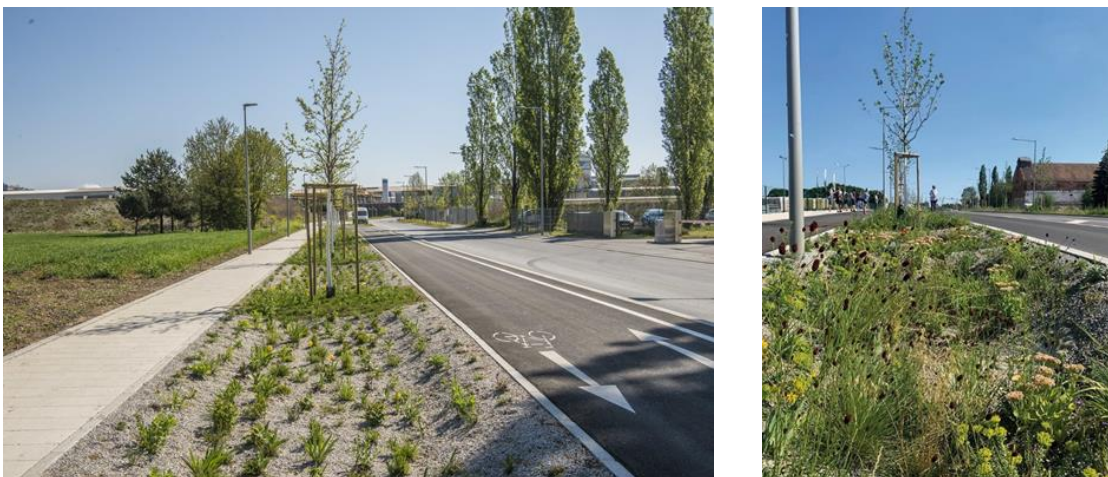
Figure 8: intentional infiltration of street water on site in Graz, Austria 15
