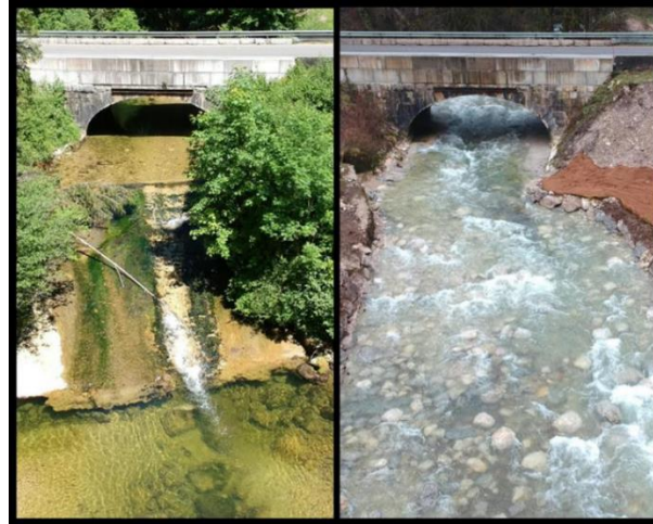
Figure 12: before and after a demolition of a barrier in France 19
