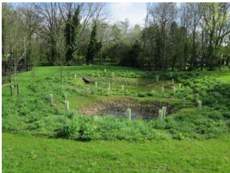
Figure 40: Infiltration Basin in Victoria Park Health Centre, Leicester 53
