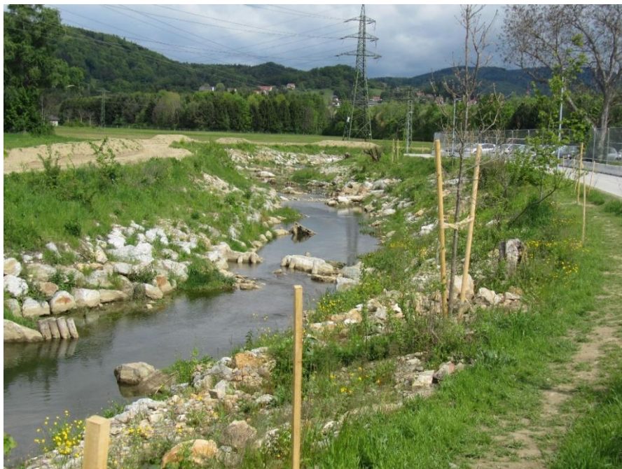
Figure 51: Restoration and flood protection project “Streams of Graz”, Graz 64
