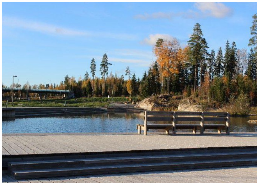
Figure 42: Wet Retention Basin in Vuores, Tampere (source: City of Tampere)
