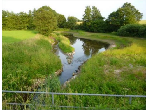
Figure 10: a nature-based sand trap near Horsdorf, Germany 17
