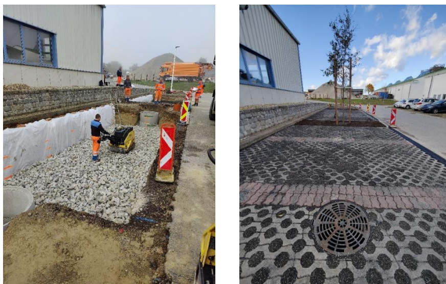
Figure 6: Sponge City concept under construction (left), the finished parking area in Wolkersdorf, Austria (right), Photo: © BAW-IKT
