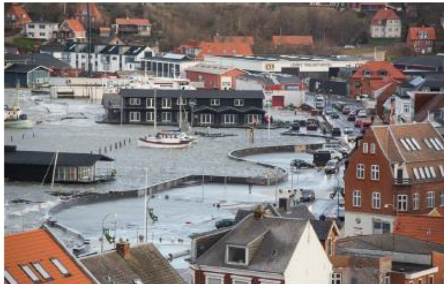
'Le Mur' protecting Lemvig harbour © Mads Krabbe
