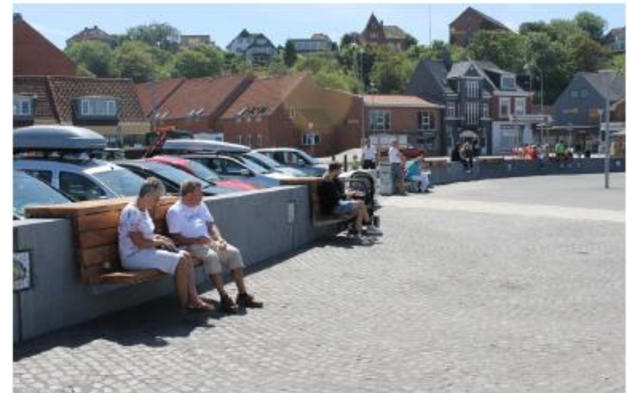
Detail of the wall © Lemvig municipality
