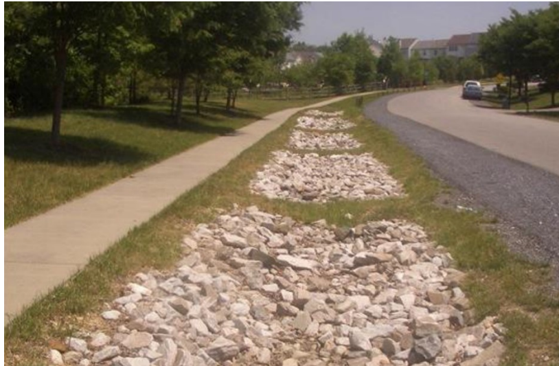
Figure 3. Infiltration trench with stones in urban area (© Andras Kis, Natural Water Retention Measure - NWRM Workshop, 2013)
