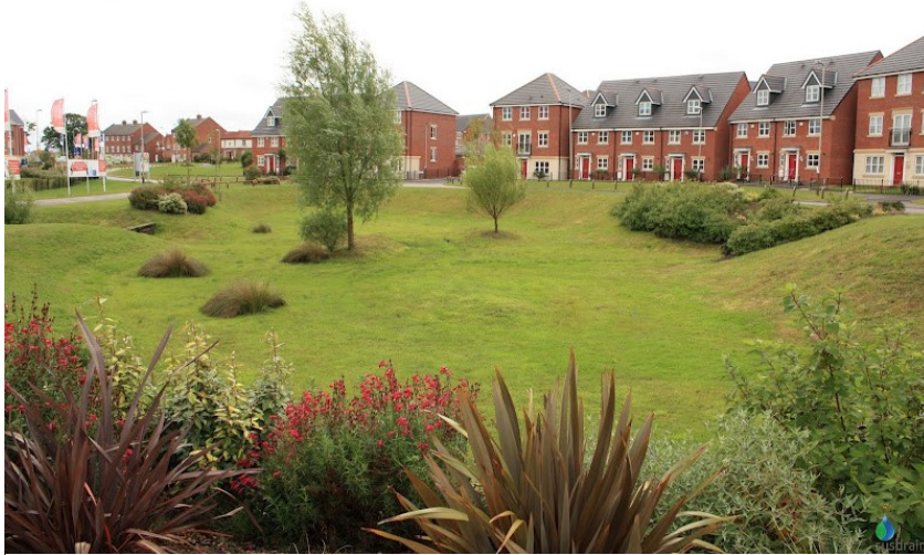
Figure 7. Detention basin (© susDrain)
