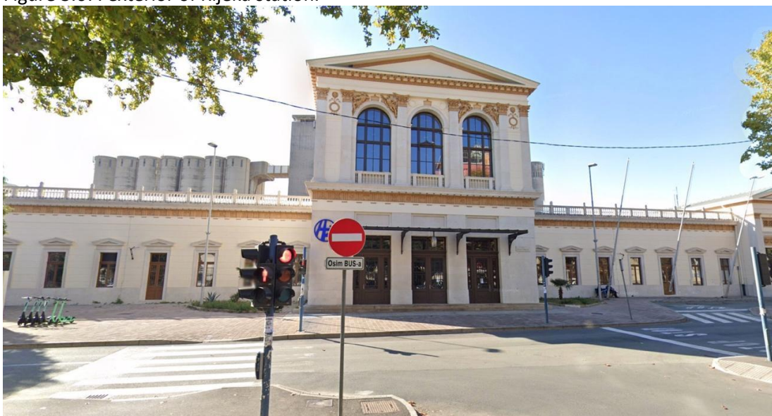
Figure 3.67: exterior of Rijeka station.
