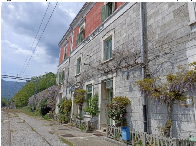
Figure 3.61: platform one and track side of the Opatija- Matulji station
