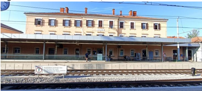
Figure 3.27: Sežana station, track side
