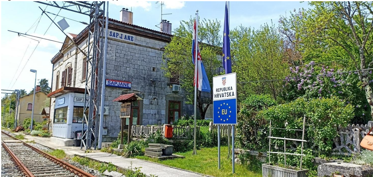
Figure 3.55: platform one of Šapjane station
