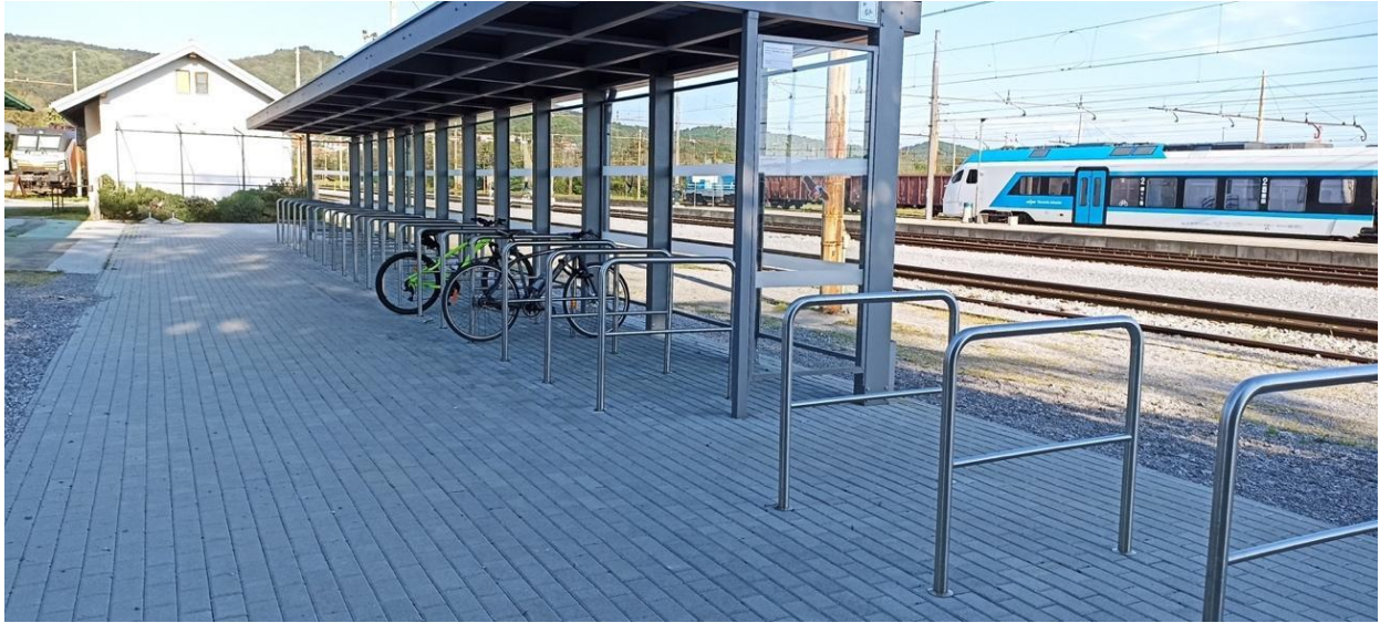
Figure 3.29: Sežana station bike park
