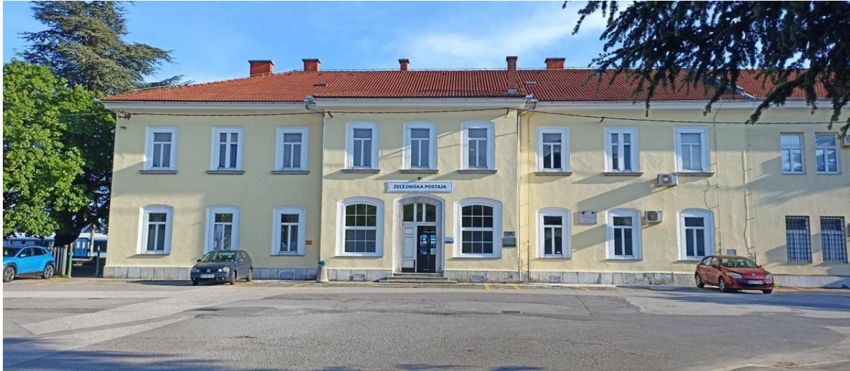
Figure 3.25: exterior of the Sežana station
