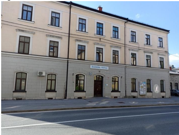
Figure 3.40: Pivka station exterior
