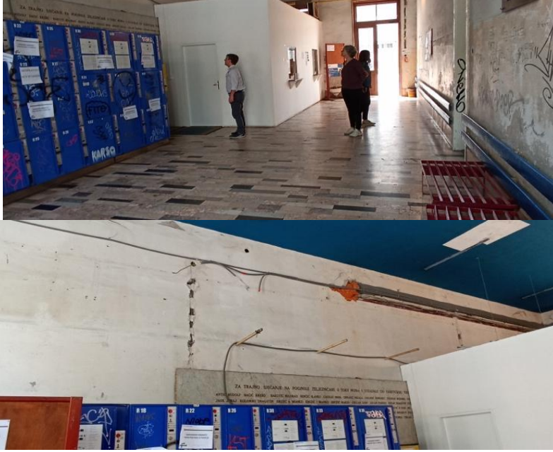
Figure 3.68: waiting room in Rijeka station and detail of the work-in-progress area
