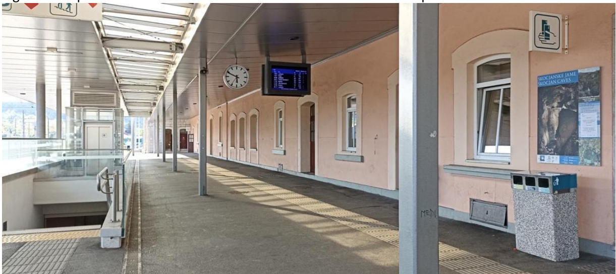
Figure 3.35: Divača station , track side.
