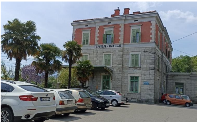
Figure 3.59: exterior of the station of Opatija- Matulji
