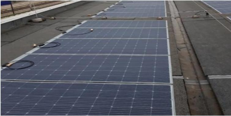
Figure 1: PV-foils on the roof of the metro station
