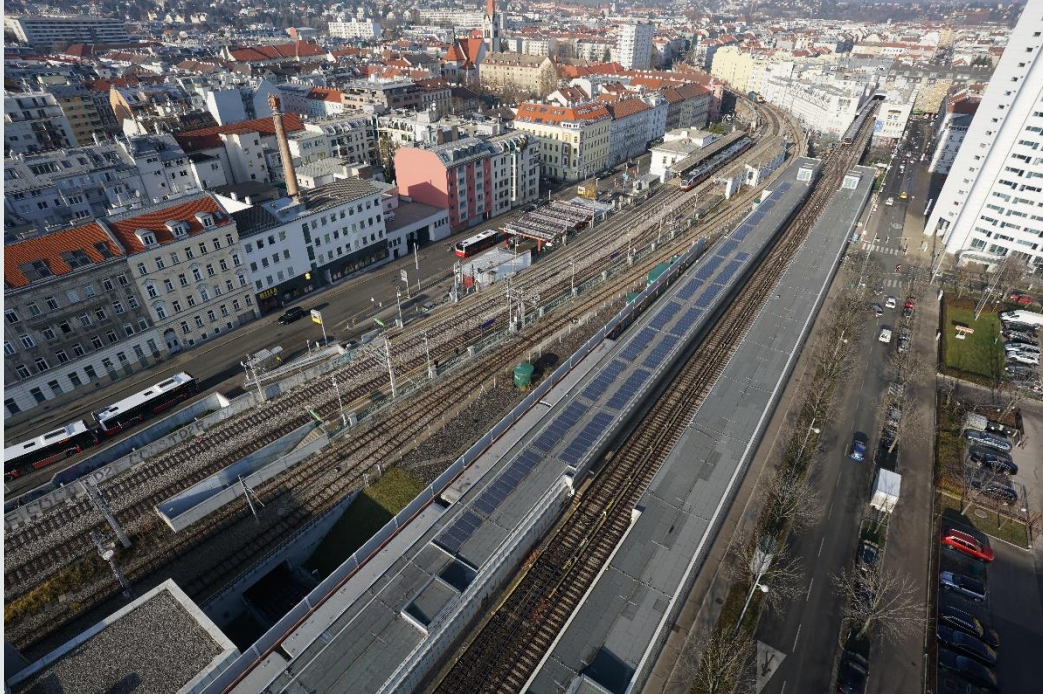
Figure 2: Aerial picture of Photovoltaic system (05-2020), Copyright Wien Energie GmbH
