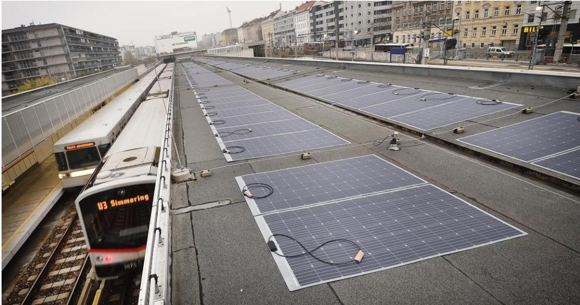
Our first pilot project was implemented in Vienna. As part of its environmental efforts, Wiener Linien launched a unique pilot project: The first-time installation of special photovoltaic films on the roof of the underground station in the Ottakring district. >> Read more [HERE!](#)
