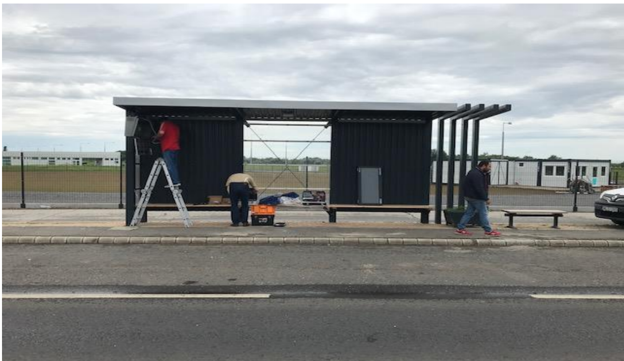
Photo 2. Panel installation at Nagykálló
