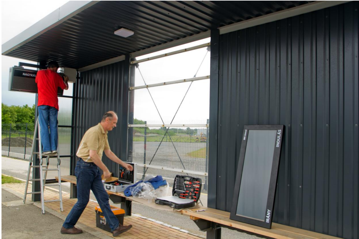
Photo 5. Panel installation at Nagykálló
