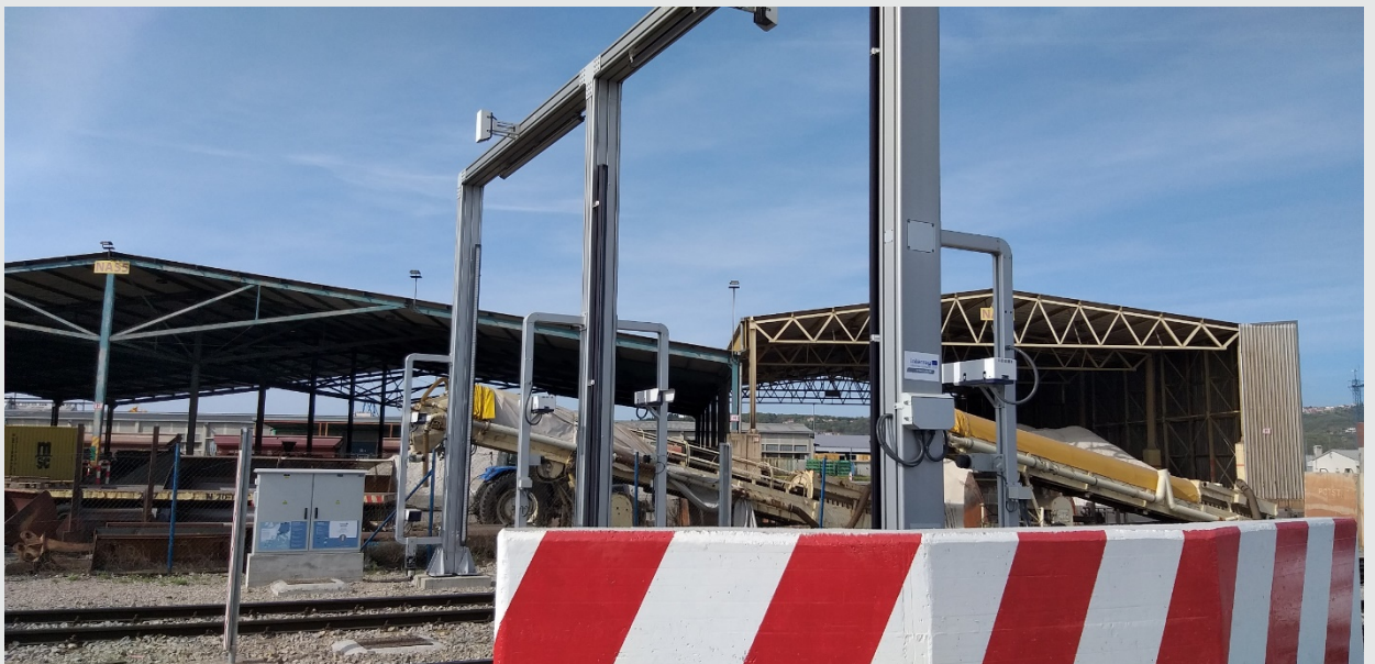
Figure 4: OCR system installed in the port of Koper (Source: Luka Koper’s archive)
