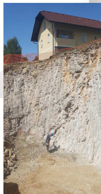
Excavation for wood chips storage
